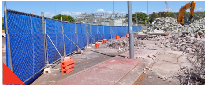
Flexshield acoustic curtains enhancing privacy and reducing noise on temporary fencing.
